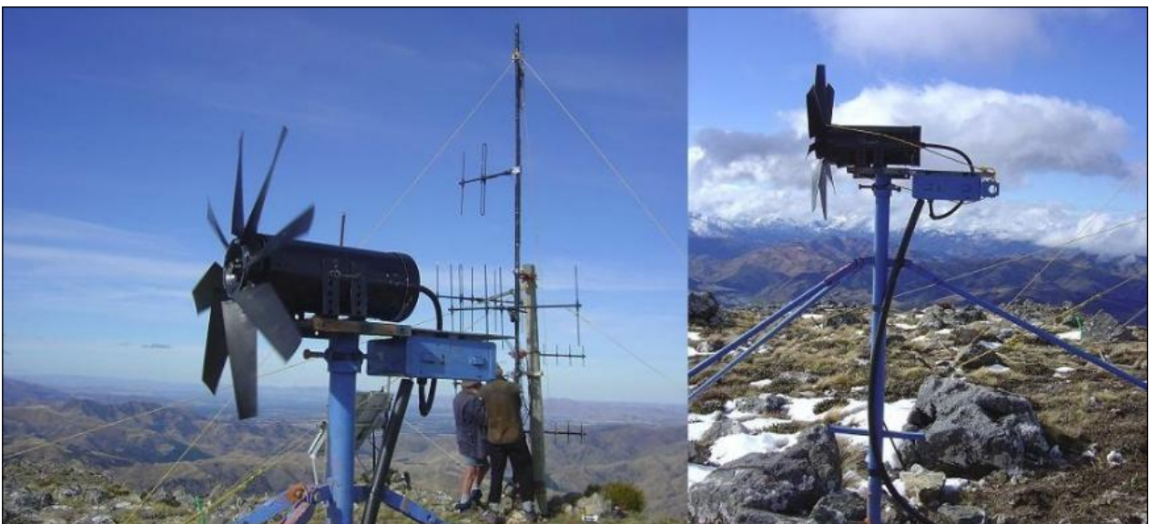
On location at Mount Noble during past repeater maintenance work
